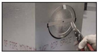
**Figure 7.9** Cut the metal retaining band and fold the sides out.
